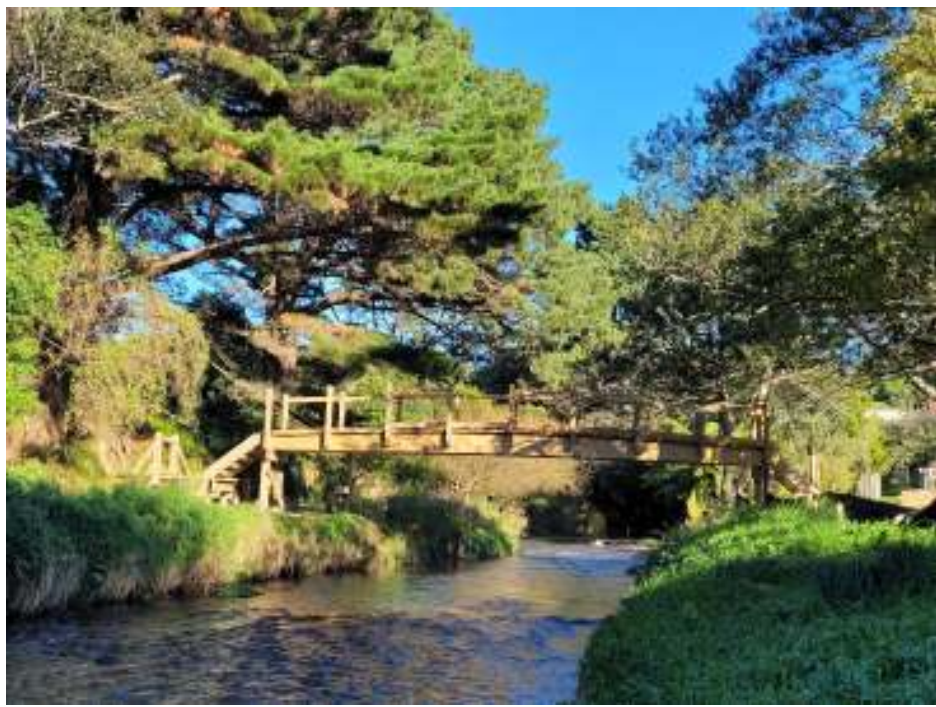
Picture of the bridge at Willowbank Park from Helen Challands
